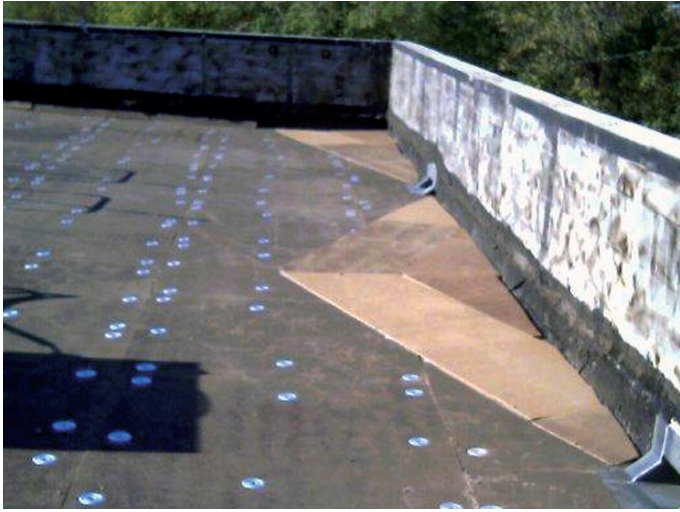
CR&R installing a 3 ply modified roofing system, Proper installation consist of using proper fasteners, drainage, insulation and ventilation are the key success of a flat roofing system
