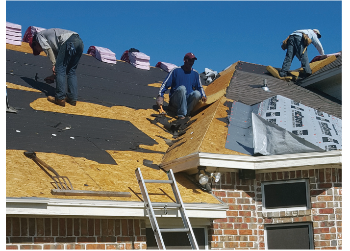
Key success of all roofing system, is using great reliable roofers, preparation of the decking, base felt, proper fasteners, proper exposure, and proper spacing.
