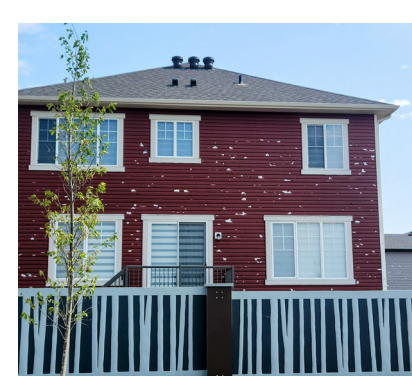
Vinyl siding windows, and fences were damaged across the city. Make sure you get line of site repairs done
