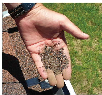
Excessive granules in your gutter or at the end of your downspouts are signs of excessive hail
